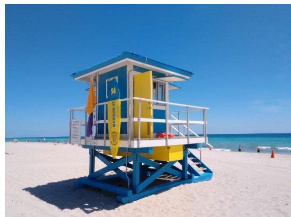
AFTER: These lifeguard stands are located within the CRA District.
